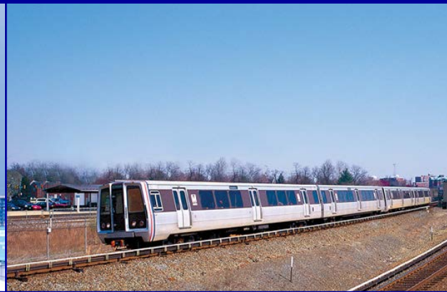
Dulles Corridor Metrorail Project
