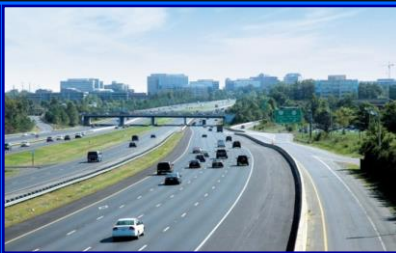
Dulles Toll Road
